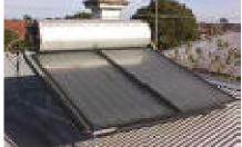
Fig. 3. Solar Flat plate collector/
